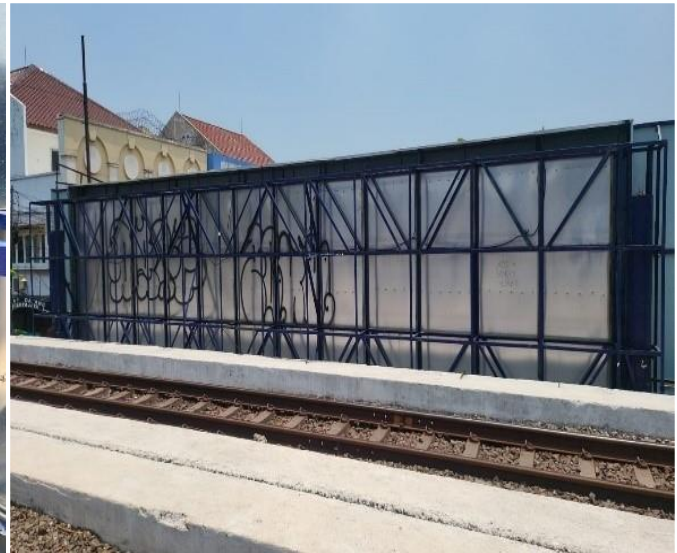
Figure 6. Construction column pipe
