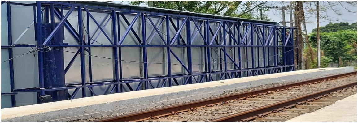
Figure 7. Picture of Installing A Silver Neon Box
