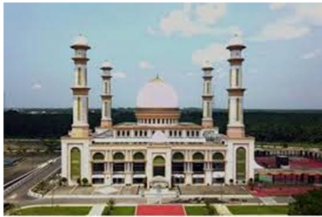
Figure 1. Exterior View of H. Achmad Bakrie Grand Mosque as a City Landmark.
